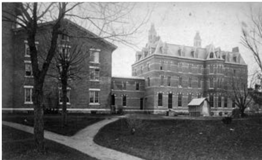
The 1878 addition adjoined the rear of the 1862 building, but was not completed as designed.
