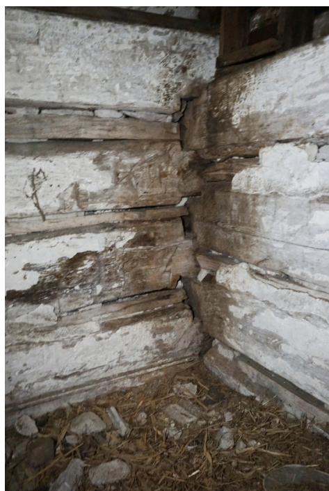
The Notter Cabin, rear ell (above), and interior view showing log construction.
