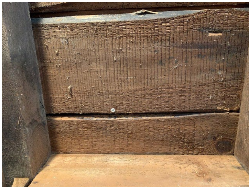
Interior wall of South Family Wash House (1823) exposed during 2019 repairs. Note the vertical saw pattern made by an up-and-down, sash- (not circular-) type saw such as the one at the Bennett's Brook mill. Courtesy of Judy Warner.
