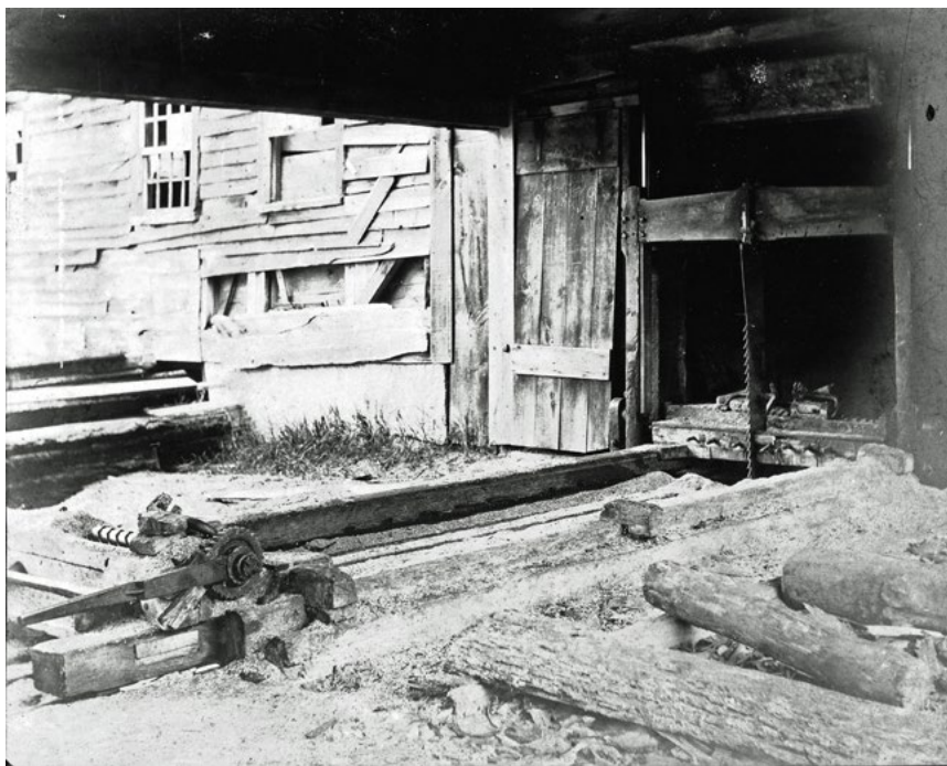
Sash saw and carriage of the Bennett's Brook Mill.
