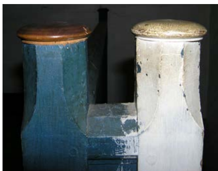
Above: Newell posts from the third floor of the Canterbury meetinghouse. The deep blue applied in 1815 is present at left. The right newell post is white, as is the woodwork on the second floor.
