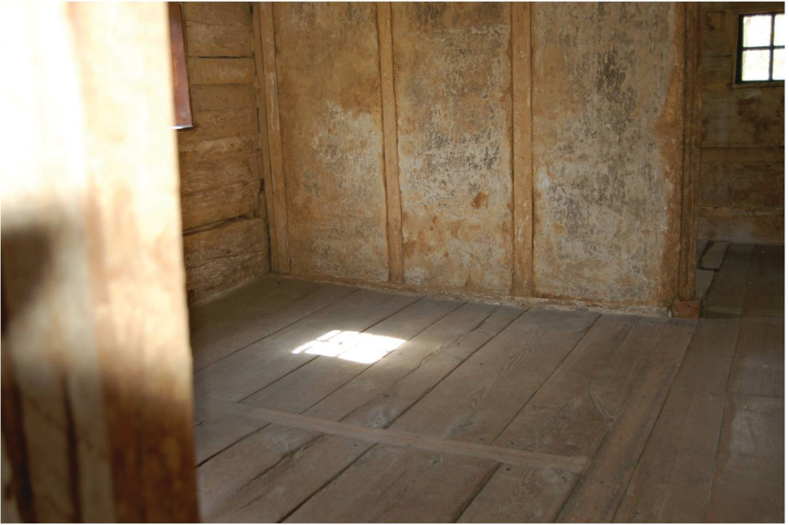
Figure 13. Second floor of Saron showing area where cell wall was removed forming larger room. Notice patch on floor where wall used to stand.
