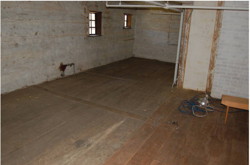
Figure 16. Second floor of Weaver's House showing floor patches where cell walls used to stand.
