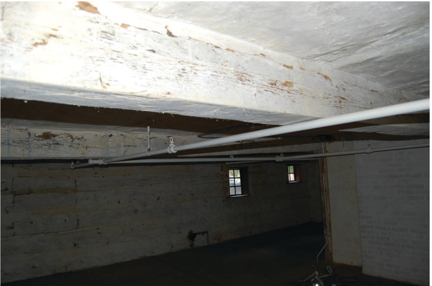
Figure 10. First floor of Weaver's House looking north showing both summer beams.
