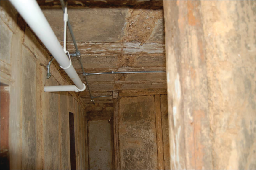
Figure 15. Second floor of Saron. Former hallway and wall have been removed. Notice where joist running along ceiling has been removed. Notice vertical grove running up vertical stud to hold lath.
