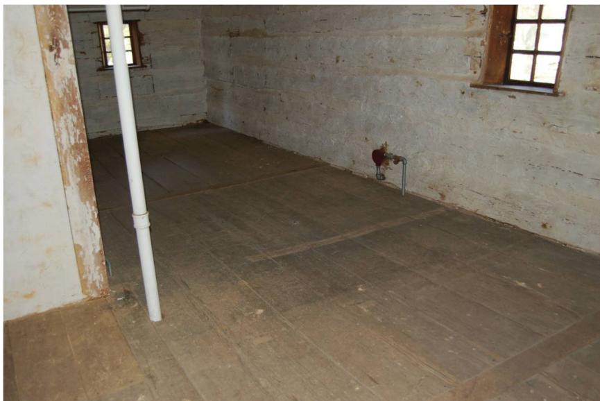
Figure 17. Second floor of the Weaver's House from the opposite angle showing floor patches denoting possible location of cell walls.
