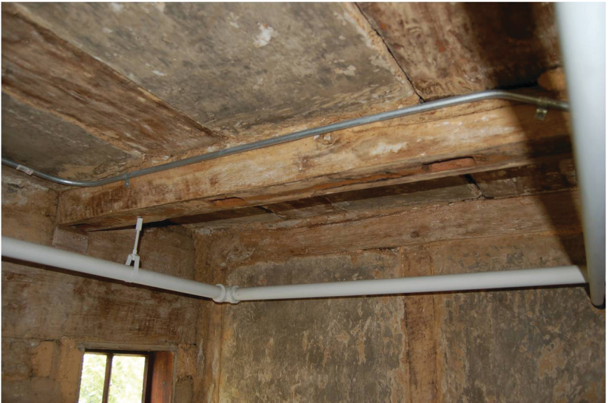
Figure 14. Second floor of Saron with ceiling joist and mortise holes where wall studs used to be. Also notice back wall with joist and stud locations.
