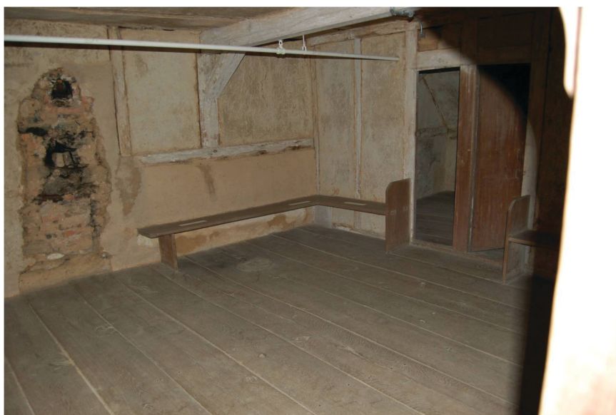
Figure 12. Second floor of Weaver's House showing both summer beams.
