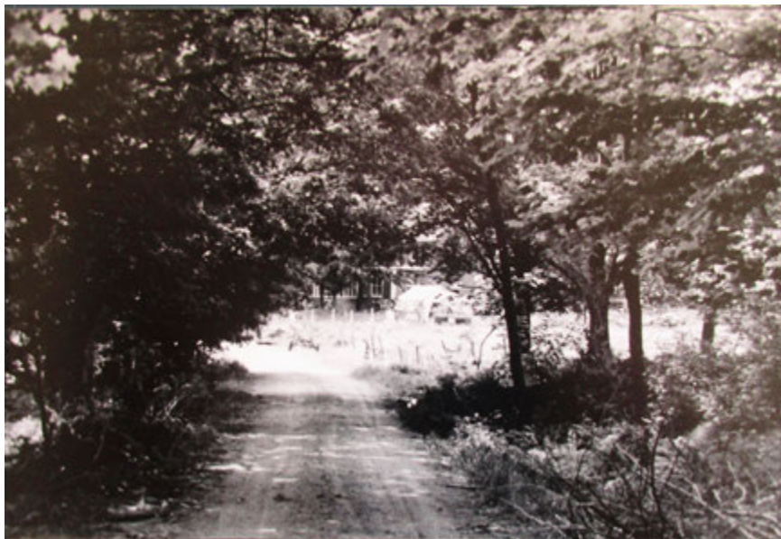
Approaching the farm from the east.
